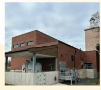
In the wake of Superstorm Sandy, renovations at Well No. 6, also known as the "Lighthouse" located at Juniper Drive, were initiated to raise the wellhead above the flood level and install a portable generator transfer switch in the event of a power outage. Here, demolition and reconstruction of a portion of the building was planned, and is now completed. A replacement pump and AOP treatment plant were installed, and are fully operational and above flood elevation levels.
